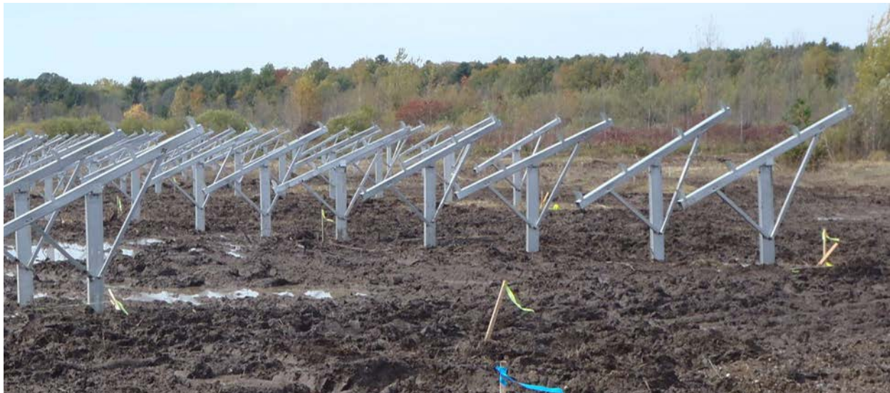
AHA Solar Farm Under Construction - Photo courtesy of Akwesasne Housing Authority
