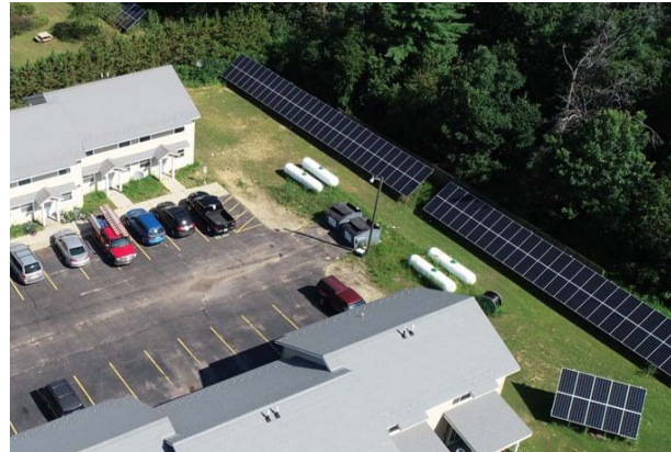
Ho-Chunk HHCD Indian Heights ICDBG Solar Project Photo courtesy of Ho-Chunk Housing and Community Development Agency
