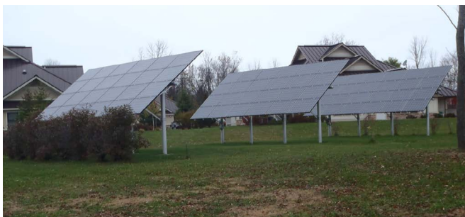
AHA Sunrise Acres Supportive Housing Solar Photo courtesy of Akwesasne Housing Authority
