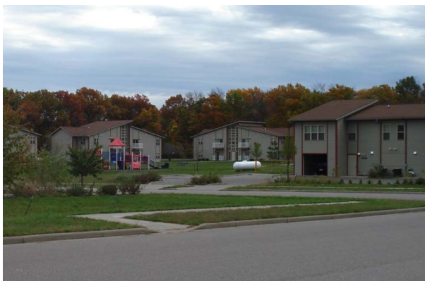
Ho-Chunk HHEDA Title VI Project - Photo courtesy of Ho-Chunk Housing and Community Development Agency
