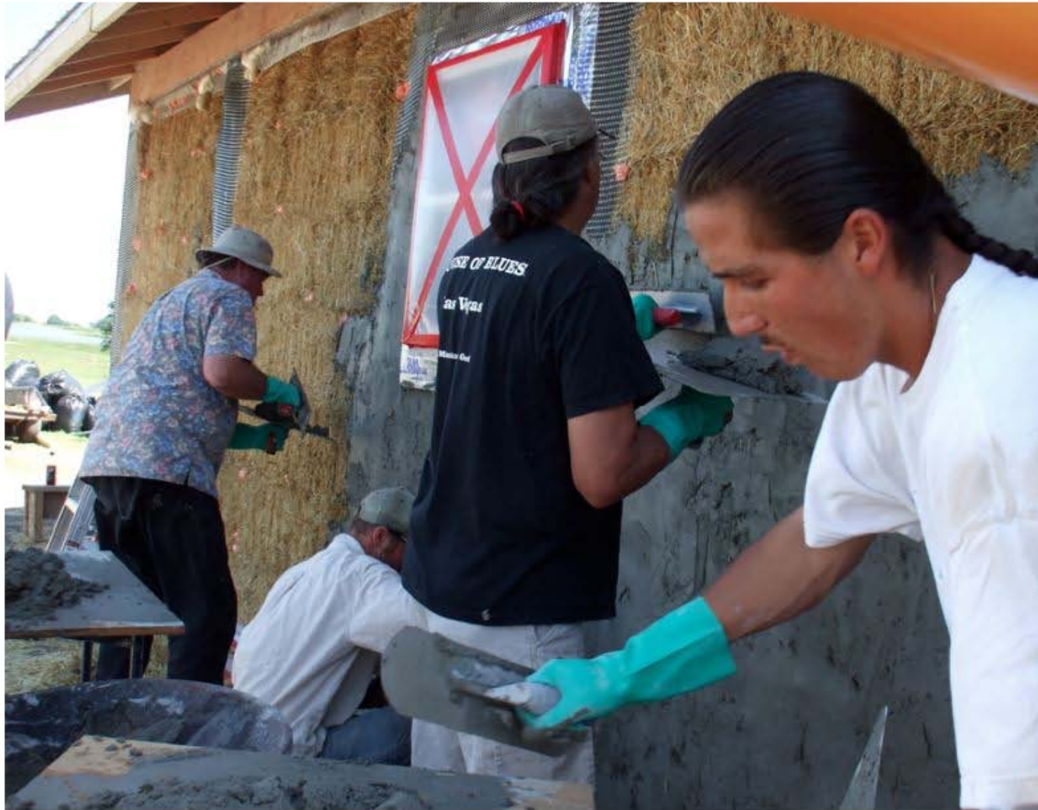
COUP SGU Buffalo Lodge Straw Bale Building Application of Exterior Plaster.
