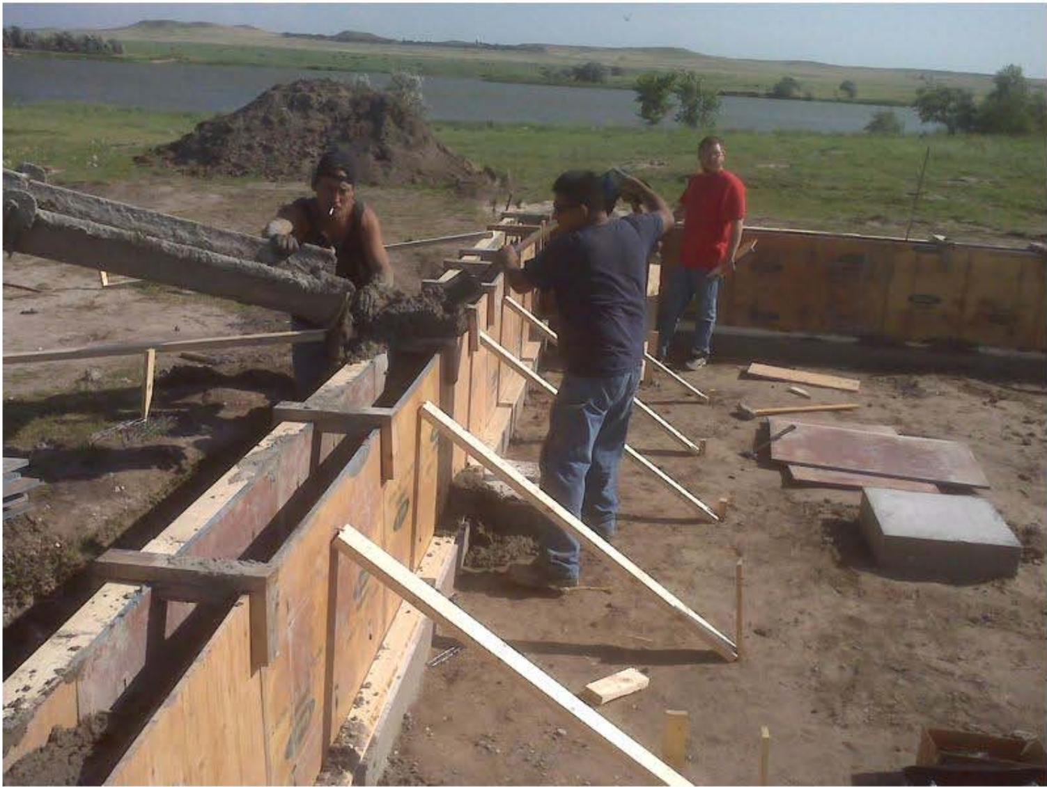
COUP SGU Buffalo Lodge Straw Bale Building pouring foundation.
