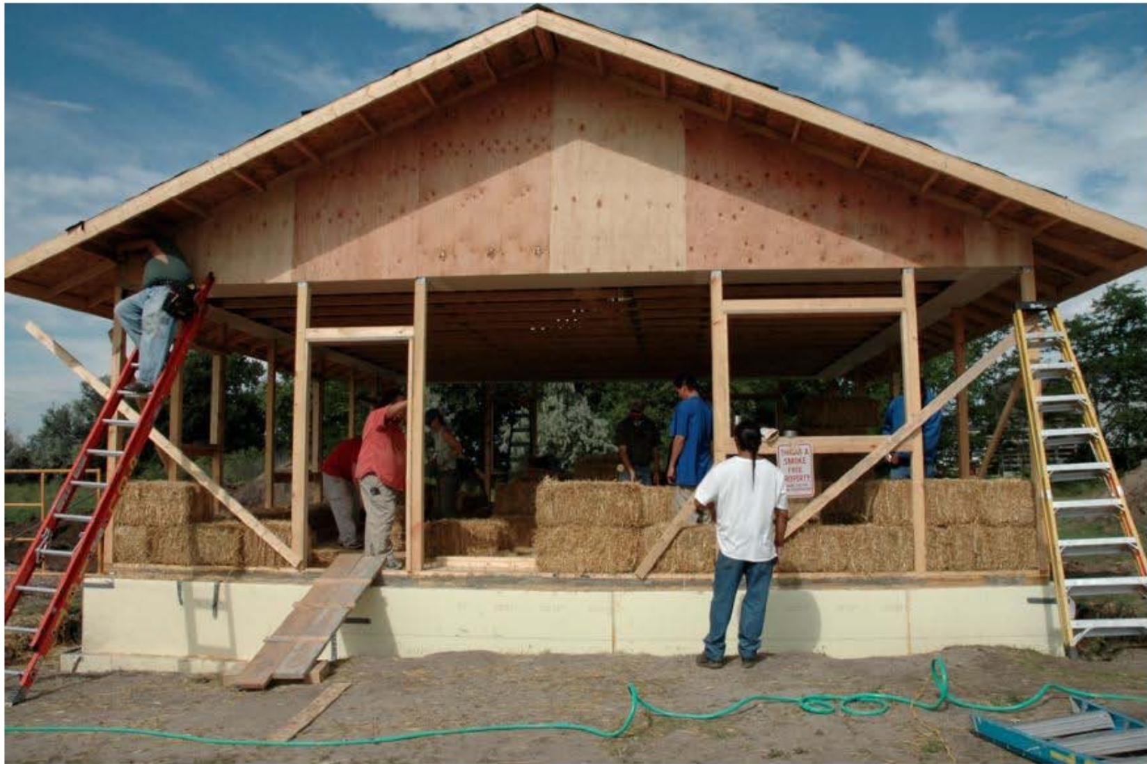
COUP SGU Buffalo Lodge Straw Bale Building Bale raising.
